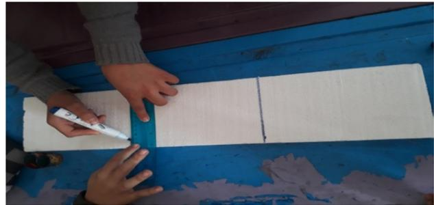
Figure 1. Measuring insulation material (foam) according to the wall size of the house
